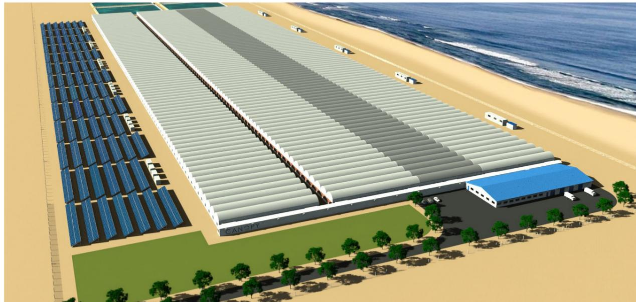
I had spent much of the previous year in Somaliland building two proof-of-concept greenhouses. My brief had been to bring together three well-established technologies – reverse osmosis desalination, solar PV power and evaporative cooling – in an off-grid greenhouse, and to grow high quality fruit and vegetables in the harshest of environments without using any fresh water, just seawater and sunlight. But I had to do this at the lowest capital cost possible.
